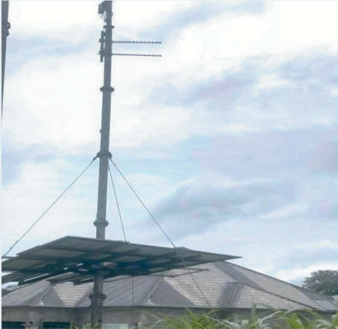
Figure D.4. Solar-powered network mass for the entire community
