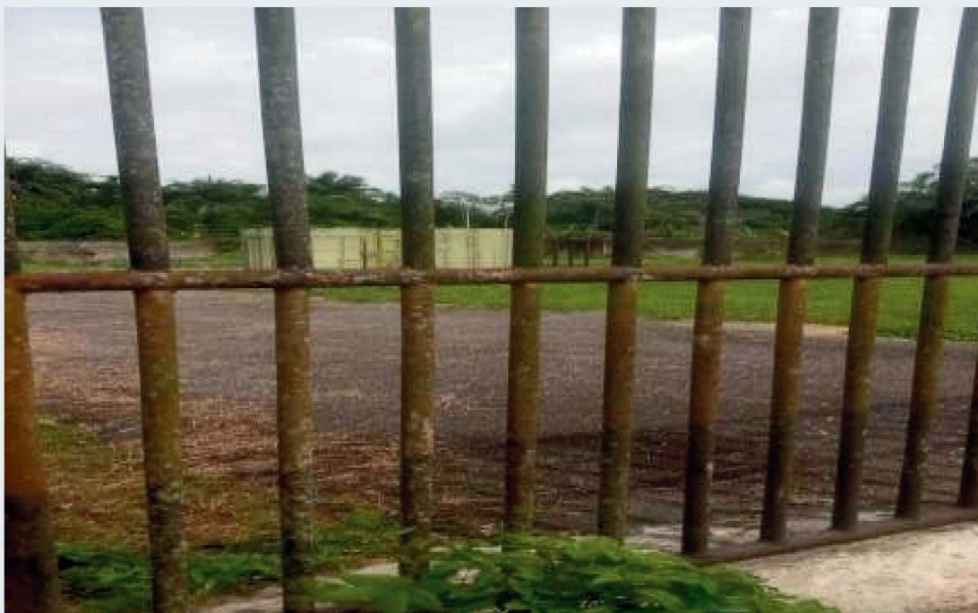
Figure E.2. Shell flow station at Imiringi
