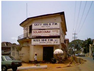
Solarcom's Freetown business office on Pademba Road. Still closed in April, 1998.
