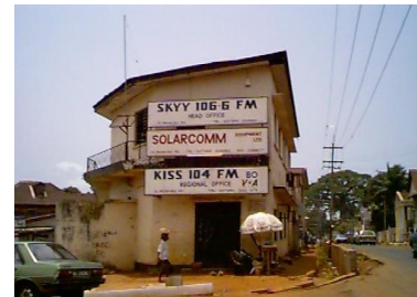
Solarcom's Freetown business office on Pademba Road. Still closed in April, 1998.
